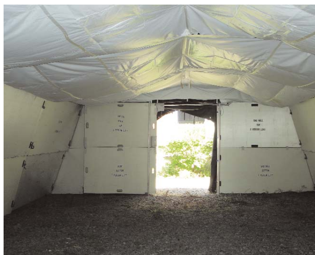
Fig. 2: MBPS installed in TEMPER tent
